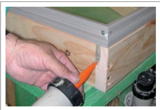
Figure C9.3.26 Application du scellant
