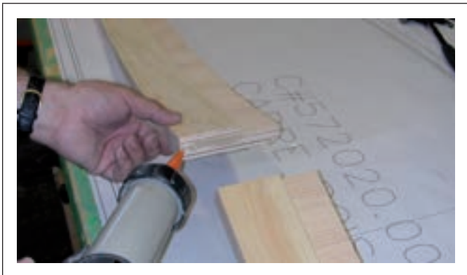
Figure C9.3.32 Application de scellant
