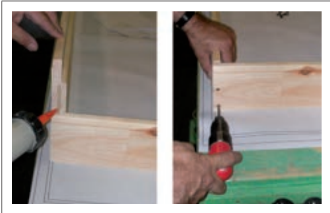
Figure C9.3.38 Pose de meneaux
