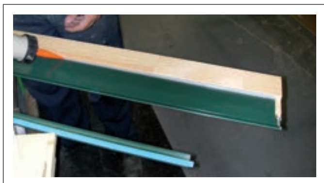
Figure C9.3.5 Application du scellant
