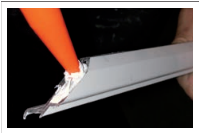
Figure C9.3.52 Application du scellant
