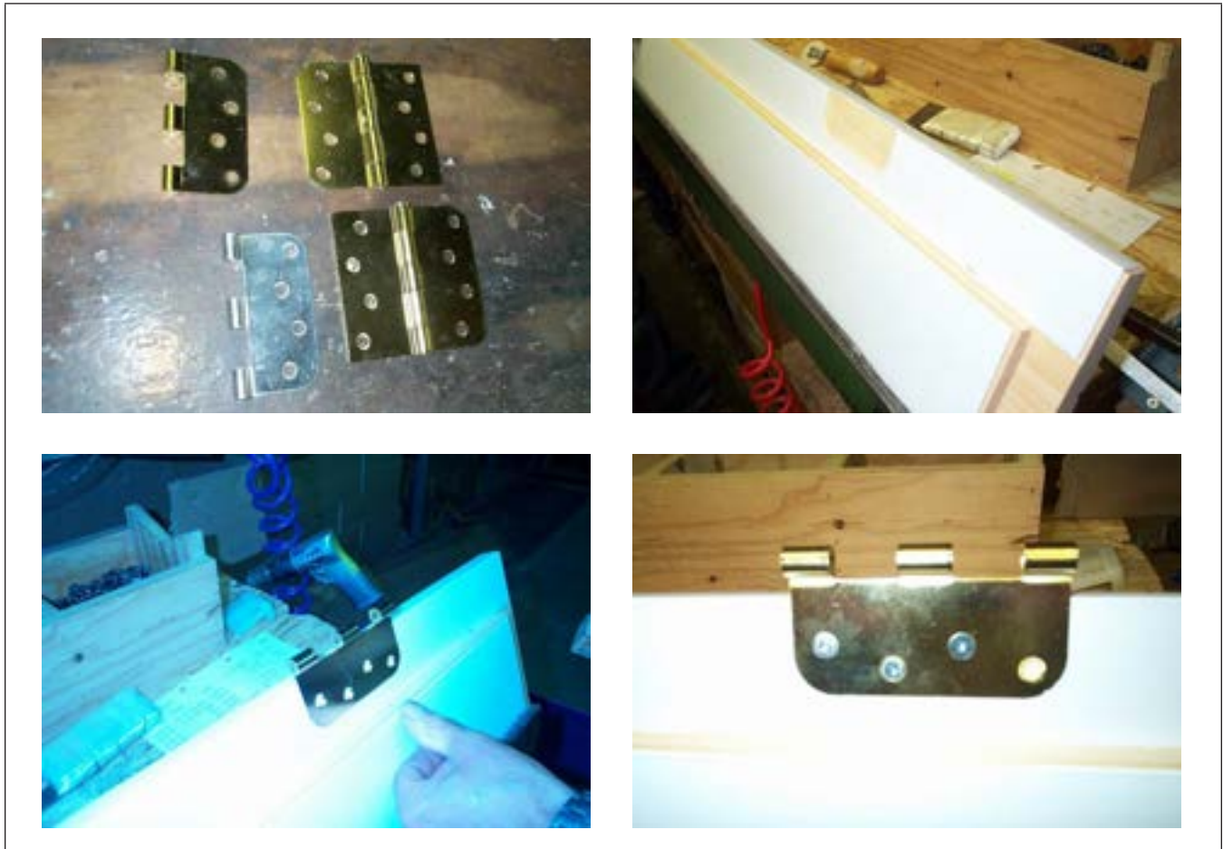
Figure 4.5.8 Installation des pentures
