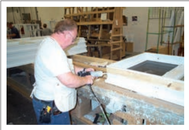
Figure 4.5.30 Pose du scellant (silicone)
