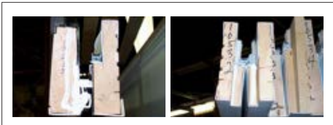
Figure 4.4.4 Pose du scellant
